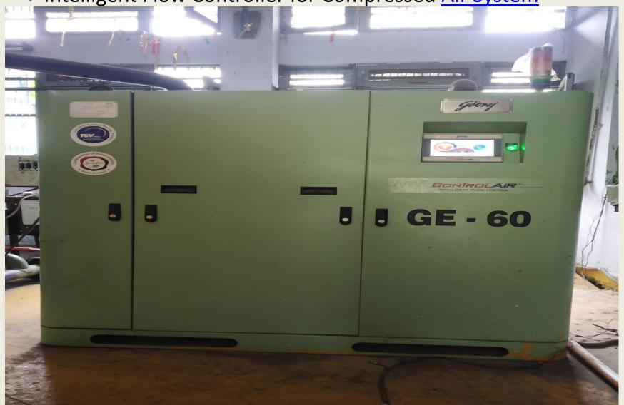
Use of Baby Compressors for individual shop in place of centralized compressed air piping system
